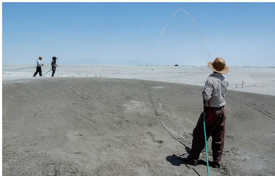
At the northern end of Lake Urmia, Sirous Ebrahimi and his team are watering sand dunes with a bacterial medium that is meant to both stimulate plant growth and form a crust that stabilizes the dunes.
